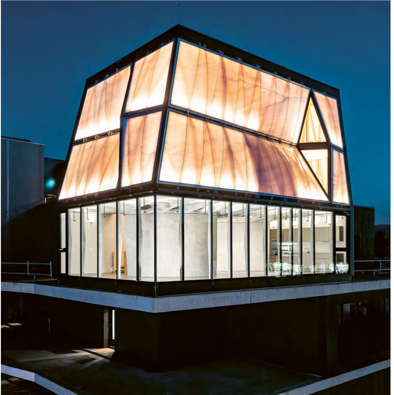
The NEST unit DFAB HOUSE at night. Photo: Roman Keller
