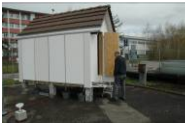
Eawag and Empa researchers use this model building to study how rainwater leaches out biocides used as antifungal and antialgal additives in facade paints and renders.
